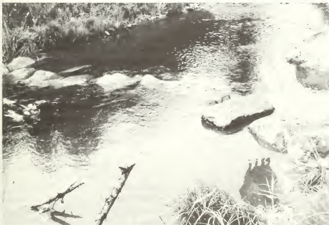
The BLM in Idaho created this rock dam to improve spawning and rearing fish habitat in a riparian area on public lands.
